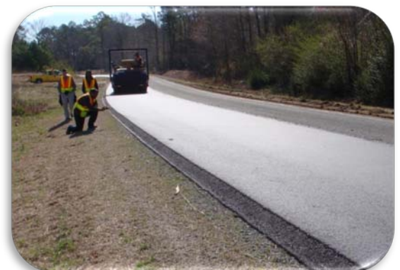
Safety Edge Installation: North Carolina 2011
